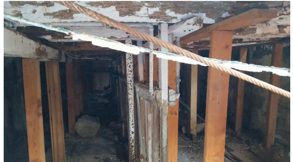
Photo 11: Interior lower level of Gurski Barn
