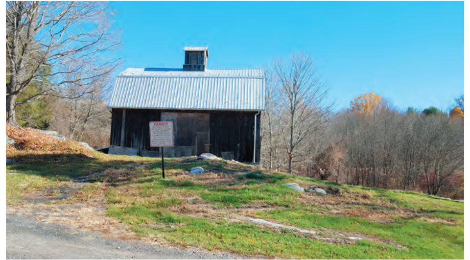
Photo 6: West Elevation of the Gurski Barn
