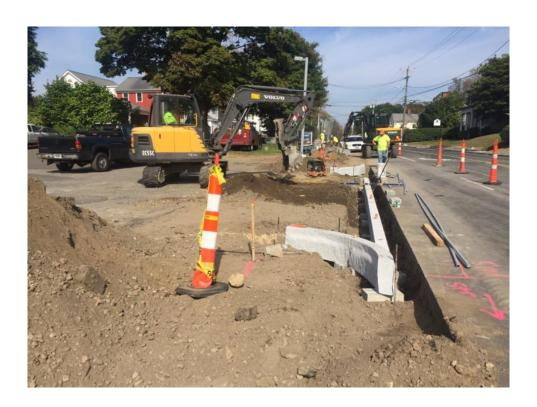
Eversource has completed moving its wires over the new poles. Charter is scheduled to move its cable off the old poles to the new, followed by Frontier. The granite curbing and new driveway aprons have been installed on the east side of Federal Road from the Shell Gas Station to the northern boundary of Phase 1, which is 839 Federal Road. Work has started on Station Road, Superior Service and the Mobil Gas Station north to the Agora Restaurant.
